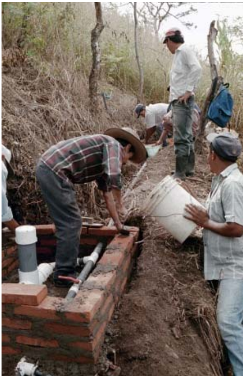
Villagers building a brick housing for their CTI 8 Chlorinator.
