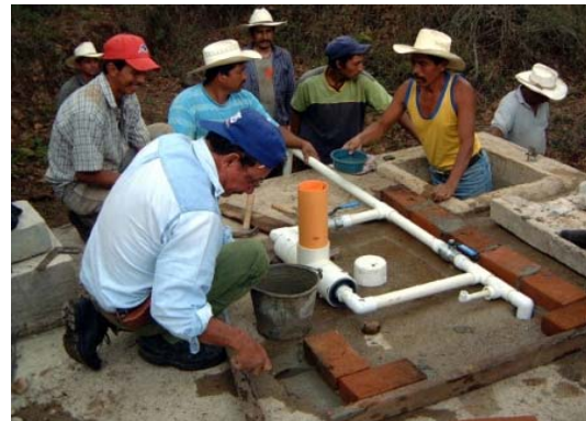
A tank-top installation in progress.
