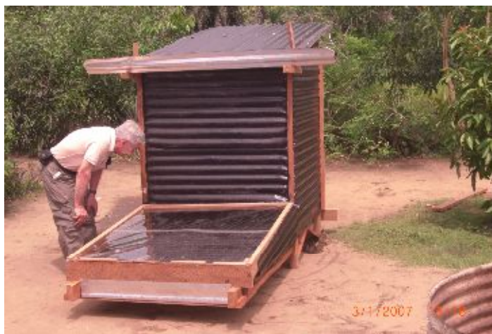
Ed Galle designed the dryer. He inspects the dryer after the construction. Back view of solar dryer with the UV resistant plastic film which collects the energy of the sun into the dryer and circulates this through the trays to dry vegetable or fruit
